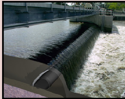
The intake chute control valve would only span the width of the intake chute (approximately ten feet).
